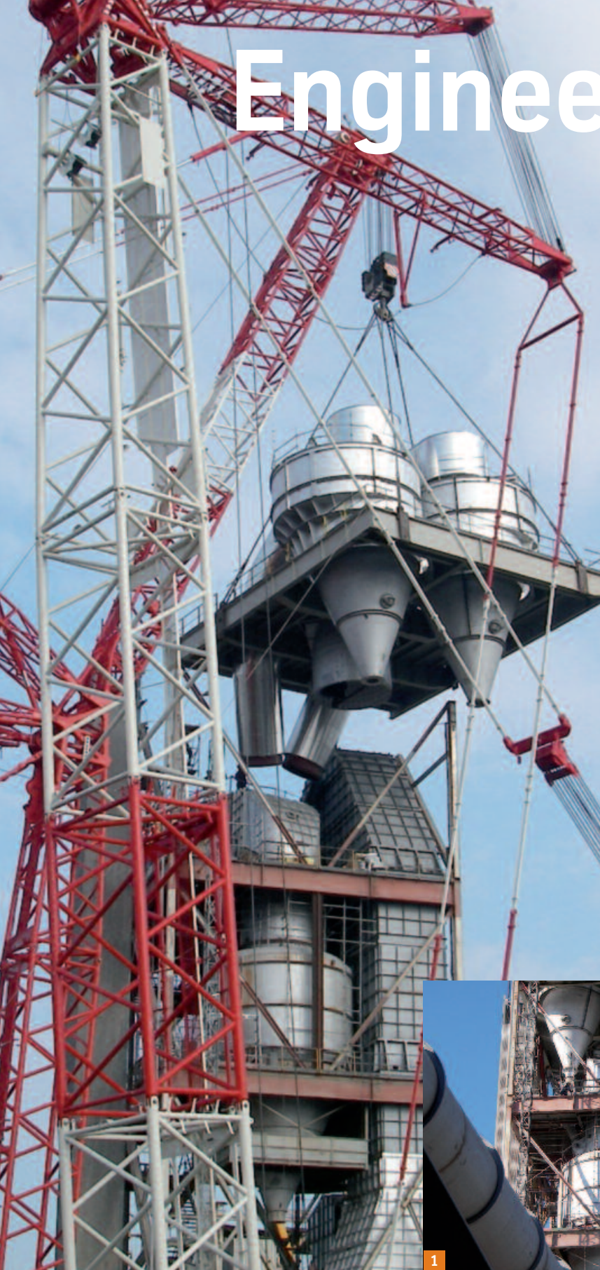
Large photo Installation of the topmost cyclone stage of a DOPOL® preheater in Spain.
