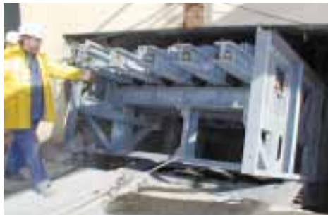
The very compact construction of the cooler permits cost-effective retrofitting, even under extreme space restrictions.
